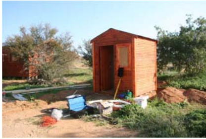
The small bathrooms get build up in the small Wendy house.
