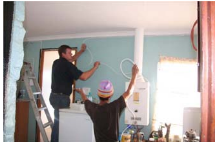
The wires for the new lights are put in.
